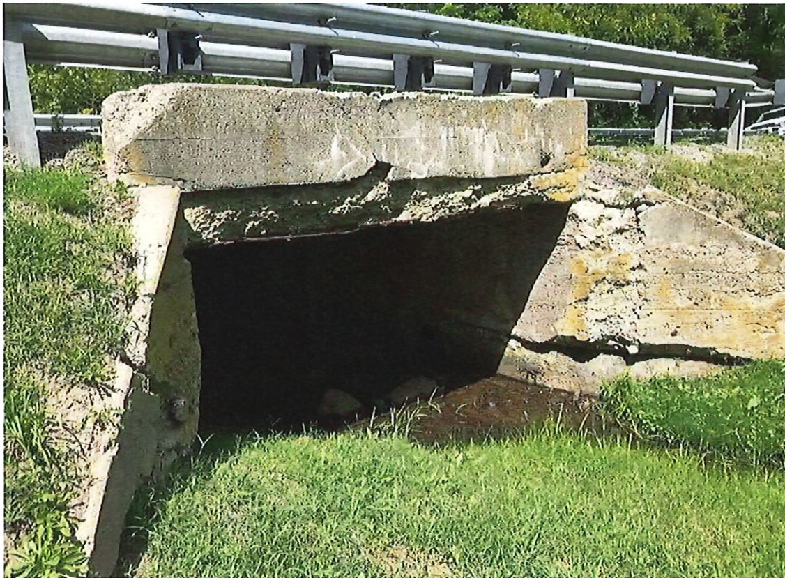
(Current picture of Old US 12 culvert, Sylvan Twp)
